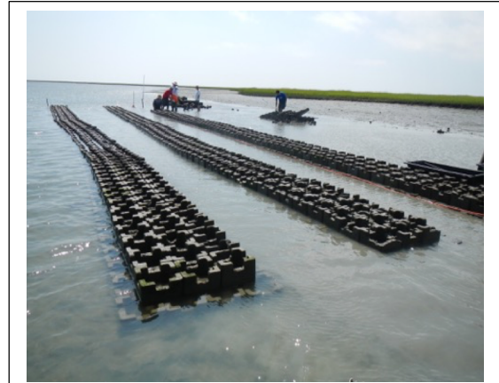
Fig. 21. Restoration experiments with oyster reefs constructed of concrete “oyster castles”.
